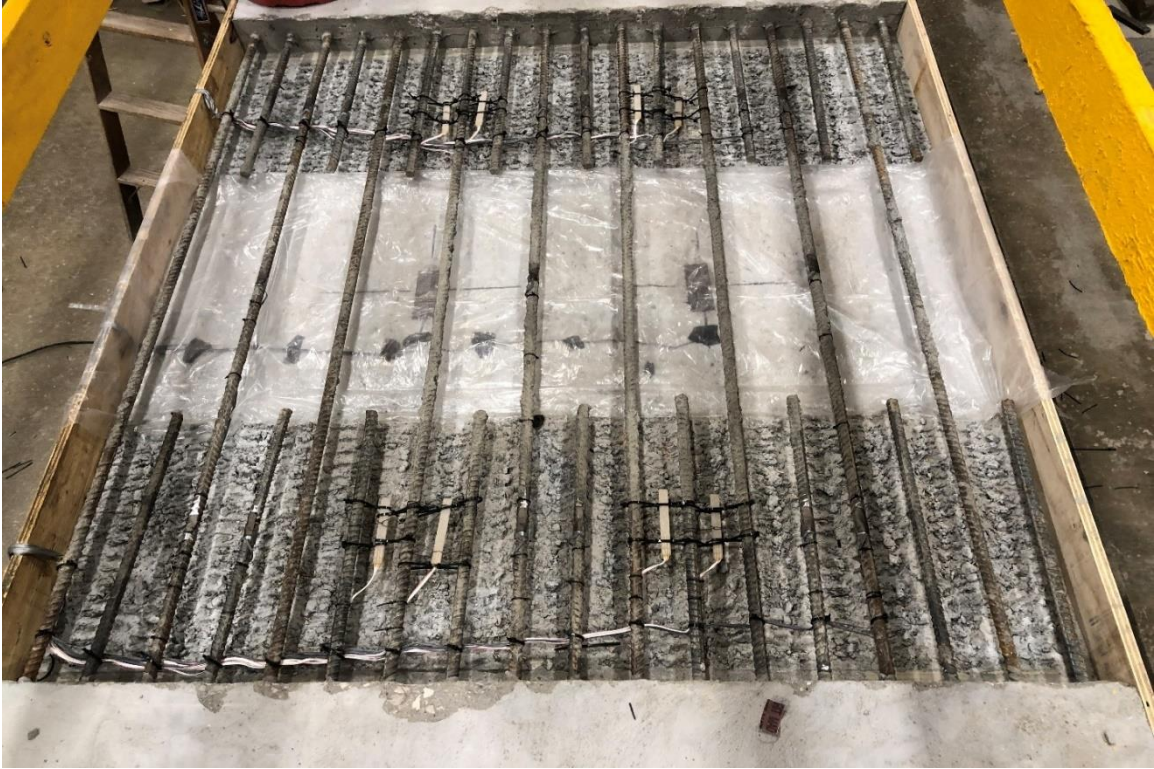
Figure 2.7 Instrumentation and debonding of the link slab portion
