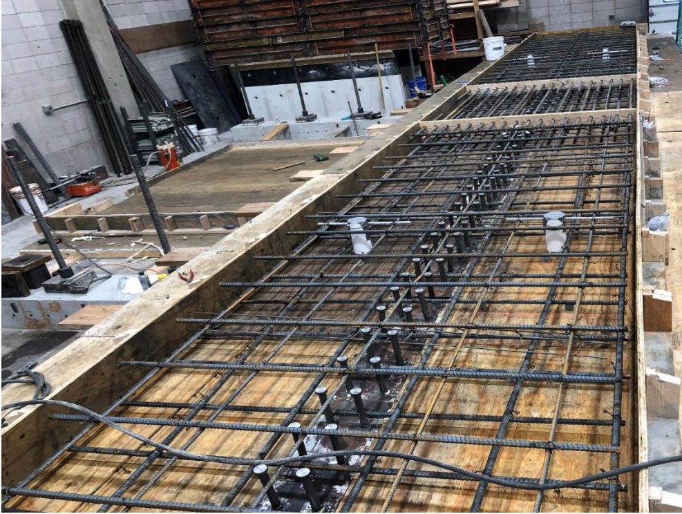
Figure 2.2 Slab reinforcement Mat
