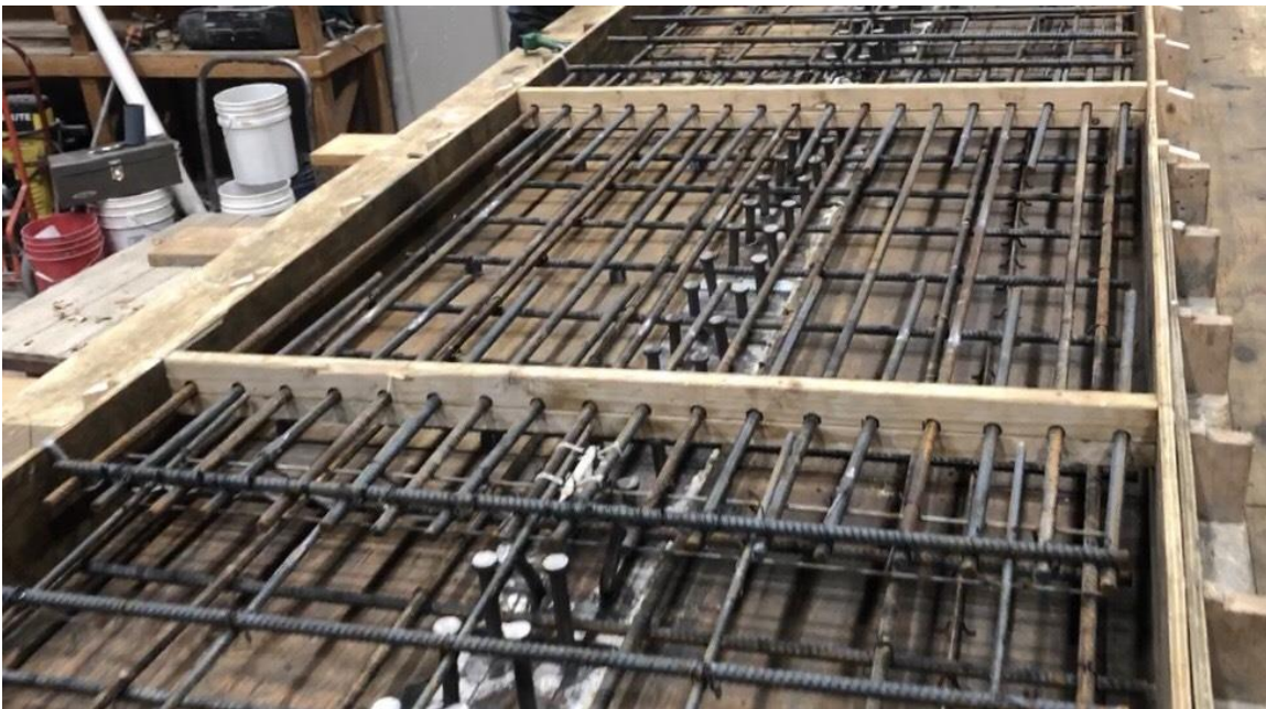
Figure 2.4 View of link slab 1 constructed in the laboratory
